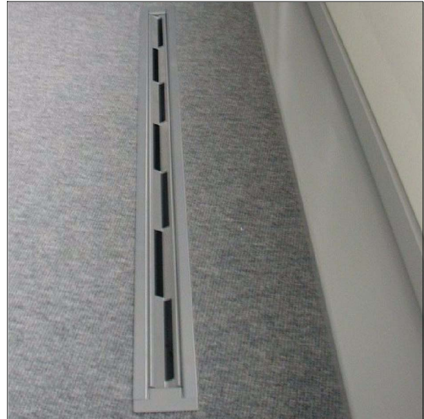
Floor-mounted linear diffuser type LDU 30/1/..., installed
